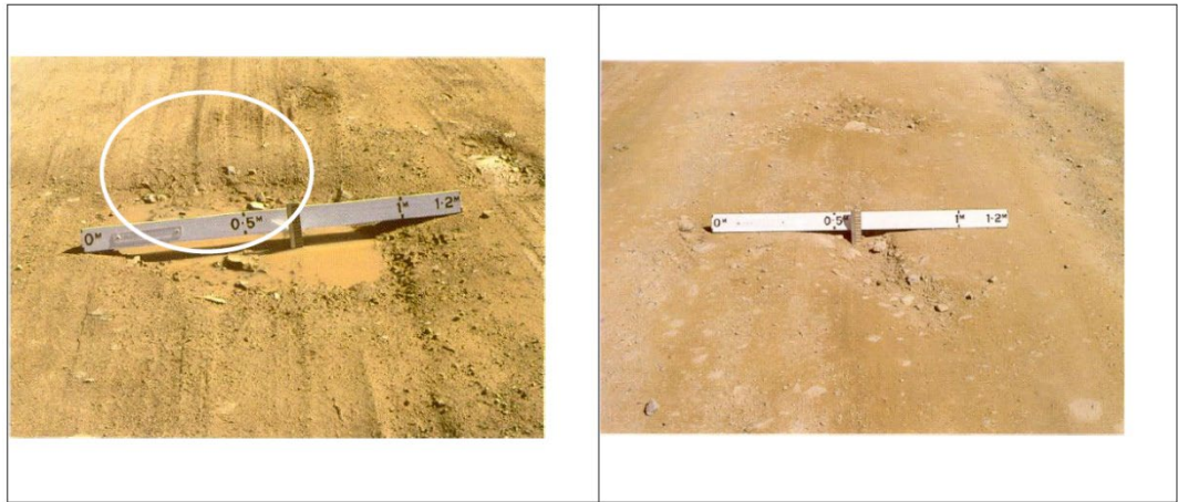
Gravel Road Pot-hole Defect
