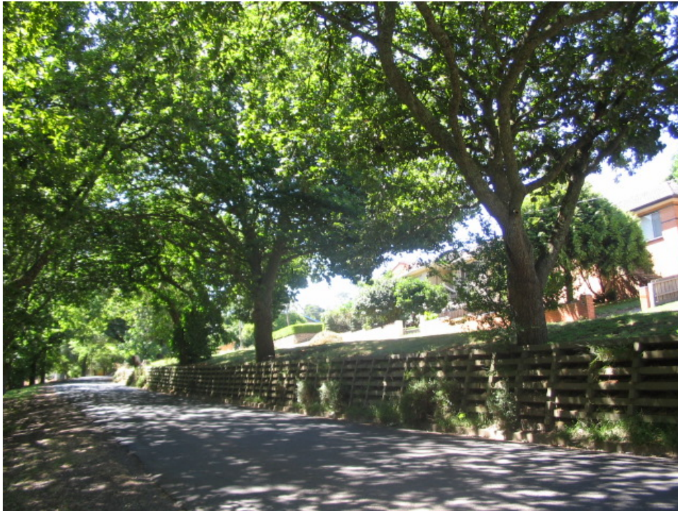
Figure 19 – Concrete crib retaining wall on east side of Oak avenue
